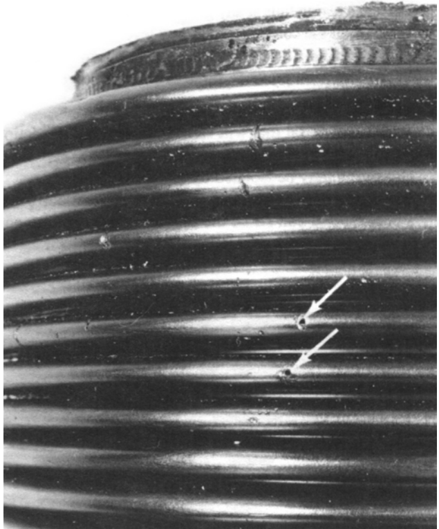
Figure 24—Pit-type Corrosion on 18Cr-8Ni Steel (Type 316) Bellows
